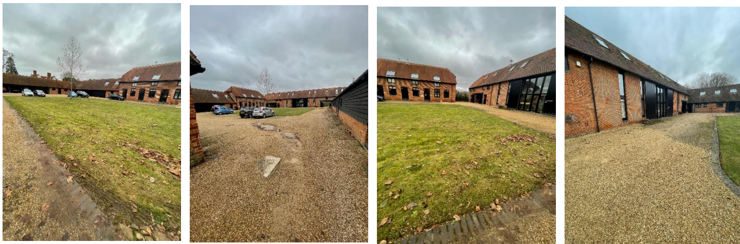
Manor Farm Development as an excellent example of the development of traditional farm buildings.
